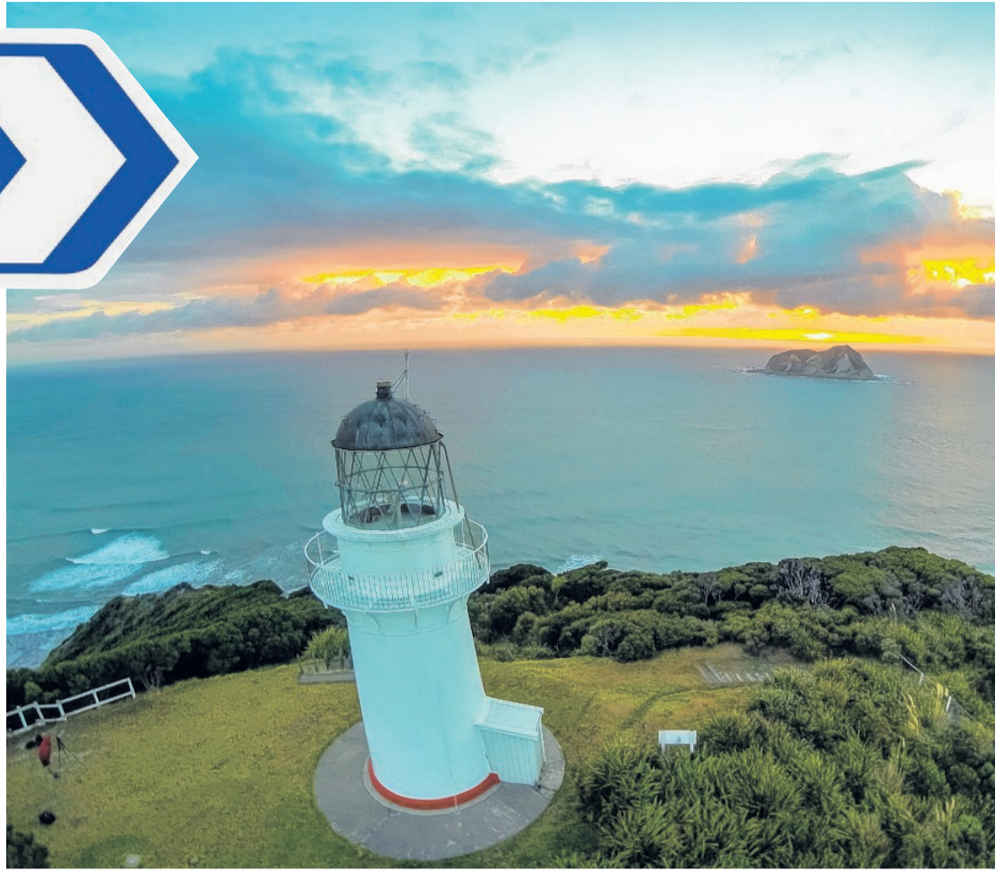
The East Cape Lighthouse is accessed by a walking track of some 700 steps.
