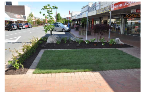
Pukuatua Street intersection upgrade
