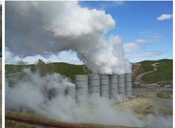
Steam field dump station being used for the first time
