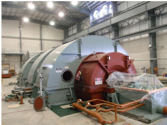
Unit 1 turbine & generator installation works
