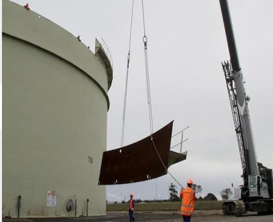
Tank demolition May-June
