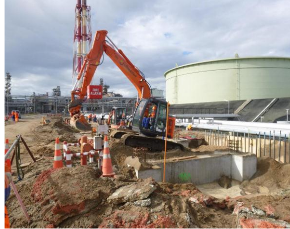
Pipe rack foundations
