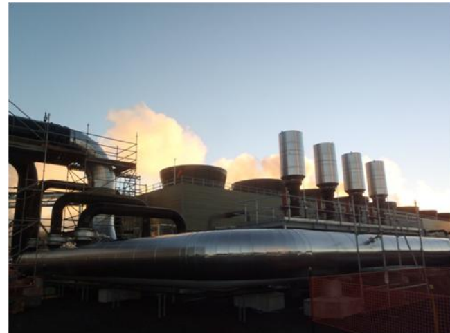
Insulation / cladding works progressing on unit 2 main steam line (cooling tower 2 in background)
