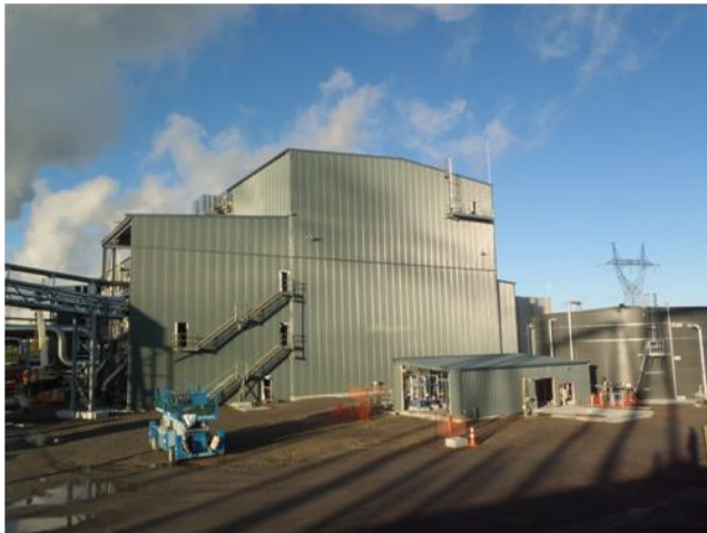
NCG extraction unit 1, turbine hall (north end) pump house and raw water tank
