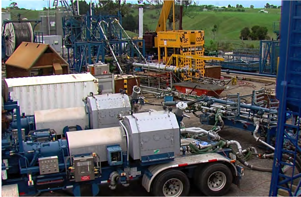
Figure 9: Hydraulic fracturing operations underway in Taranaki
