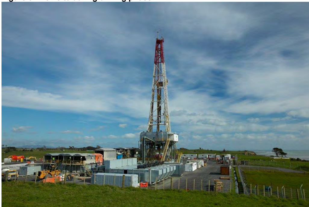
Figure 8: Well site during drilling phase
