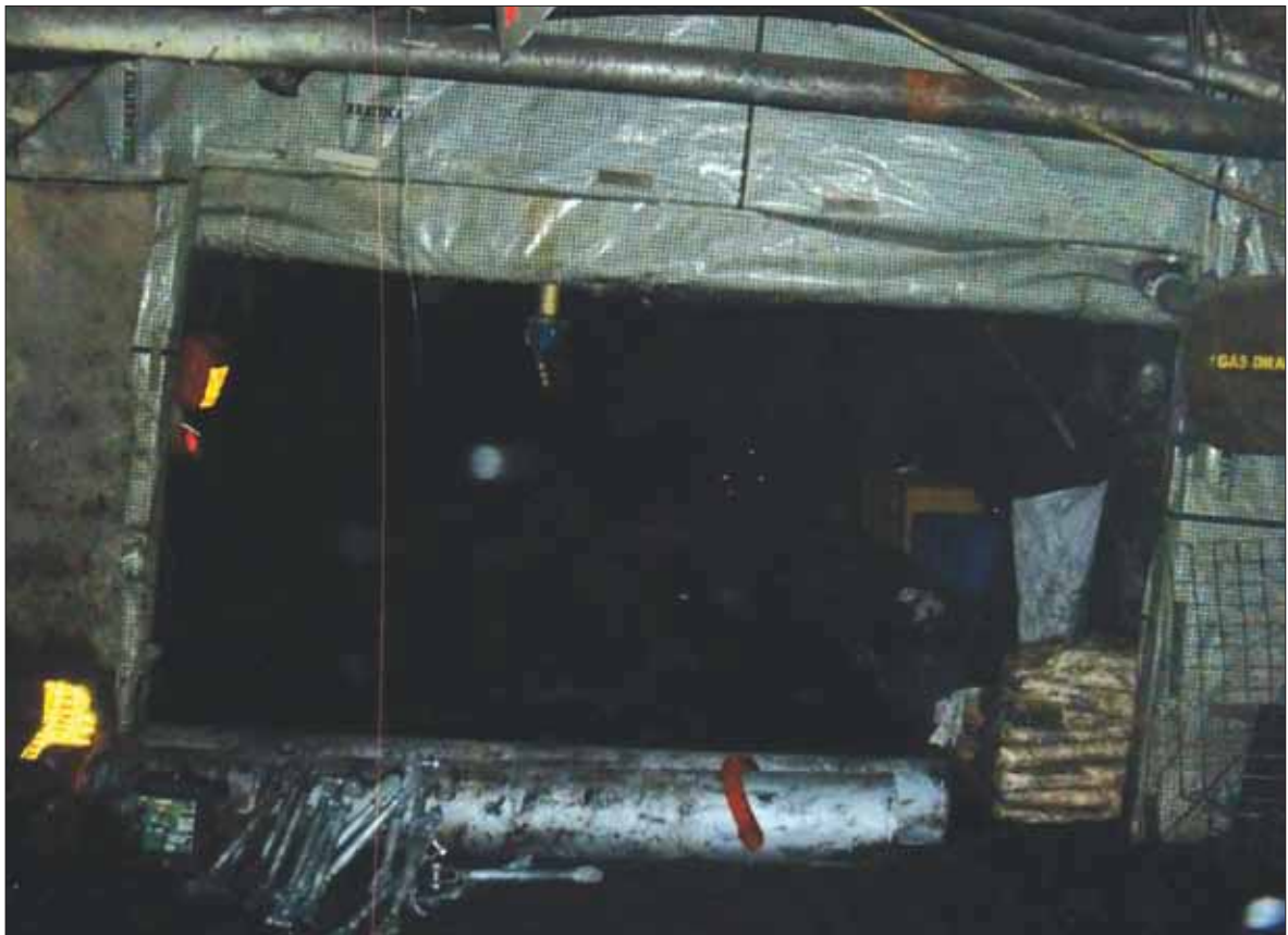
Figure 16.3: View of the upper FAB looking inside 79
