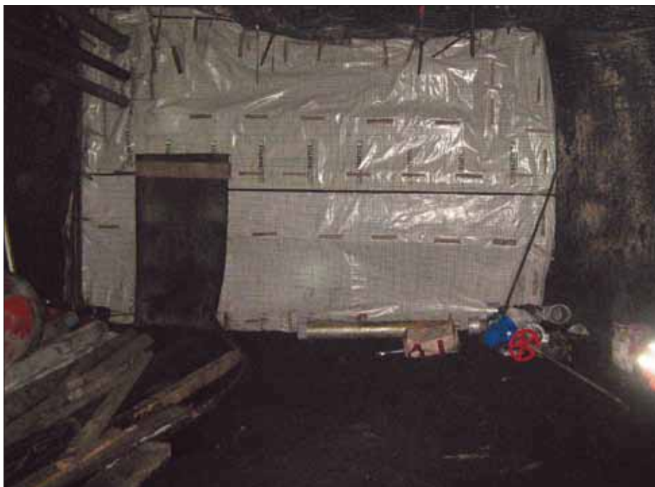
Figure 8.12: Board and brattice stopping 148
