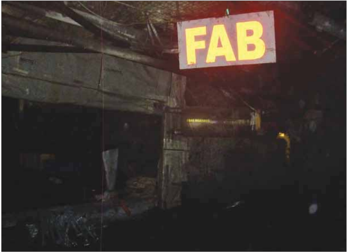
Figure 16.2: View of the upper FAB from outside 78
