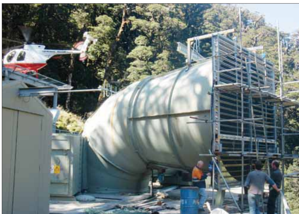
Figure 8.7: Evasé showing louvres being installed
