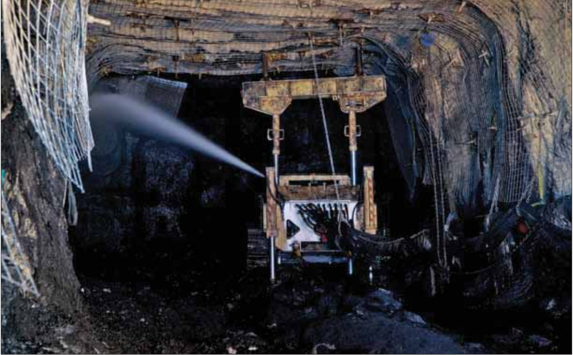
Figure 12.2: Hydro monitor at work 3
