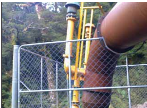
Figure 9.4: Gas riser and slimline shaft 45
