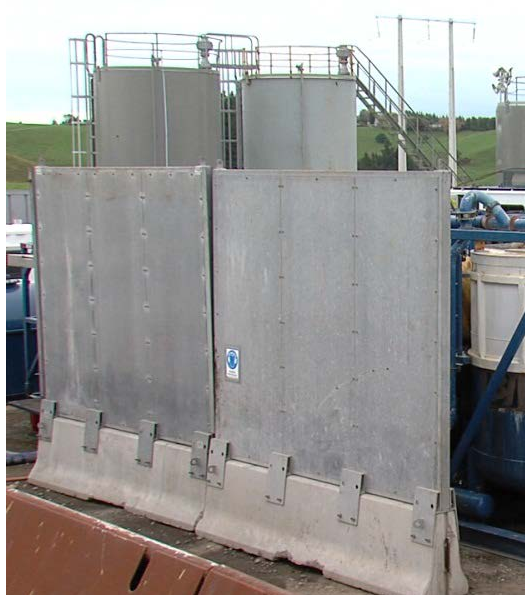
Figure 29 - Temporary noise barrier erected around wellsite equipment
