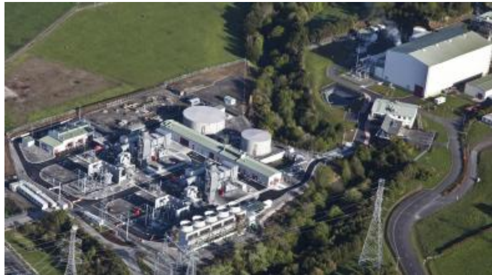
Stratford peaker and TCC power stations
