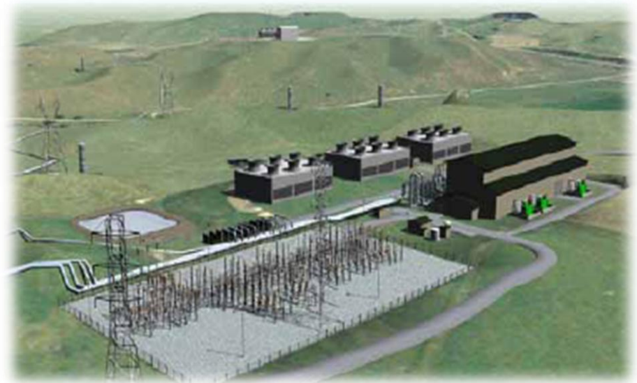
Rendition of the Te Mihi power station
