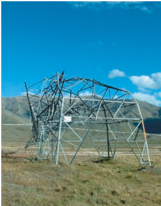
CAPTION: HVDC TOWER IN THE SOUTH ISLAND HIGH COUNTRY FOLLOWING A SEVERE WEATHER EVENT.
